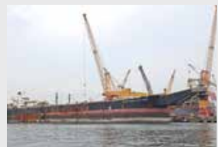
Demucking works to treat vessels for safe recycling and scrapping
