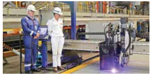
Sembcorp Marine Head of Operations Mr Wang Zijian and Norled Project Manager Mr Geir Haaland initiating the first steel cut
