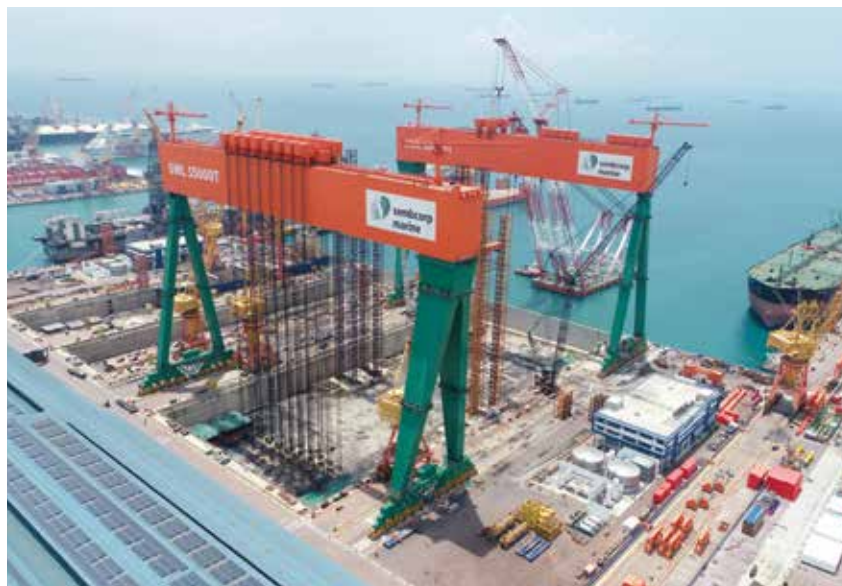
Sembcorp Marine's new gantry cranes at Tuas Boulevard Yard can hoist 30,000 tonnes in a single lift
