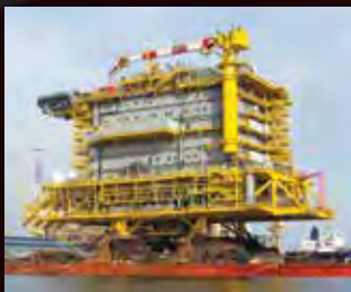
Utilities & Living Quarters Fixed Platform Topside
