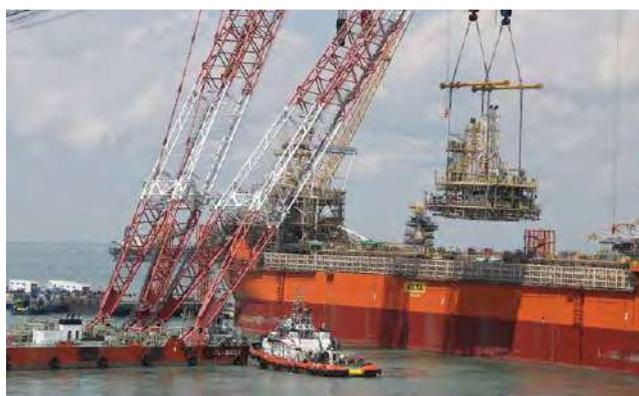
Topsides installation on a floating storage and offloading vessel which will be deployed at the Culzean field
