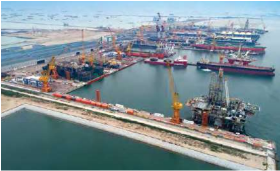
Tuas Boulevard Yard Phase II completed
