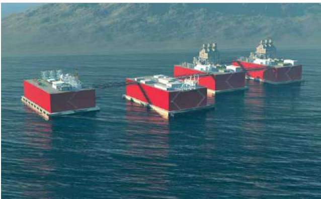
A Gravifloat solution of CCGT plants with integrated LNG storage, regasification and terminal functions
