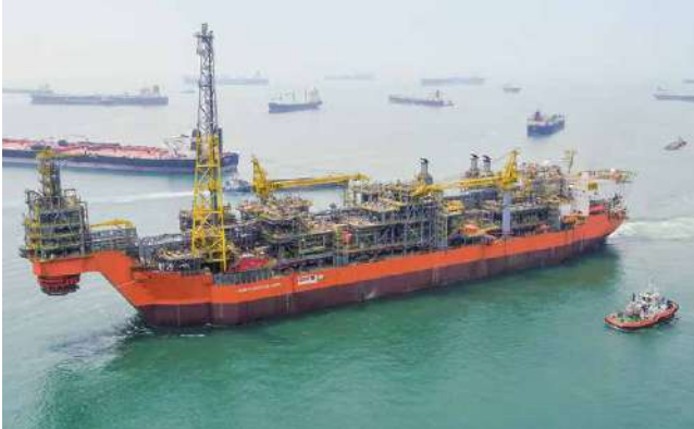
Pioneiro de Libra FPSO, Sembcorp Marine's first full EPC FPSO conversion, was delivered to joint owners Odebrecht Oil and Gas and Teekay Offshore Partners in March 2017
