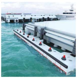
A wave energy converter system is under development to serve as an alternative eco-friendly power source for the new yard.
