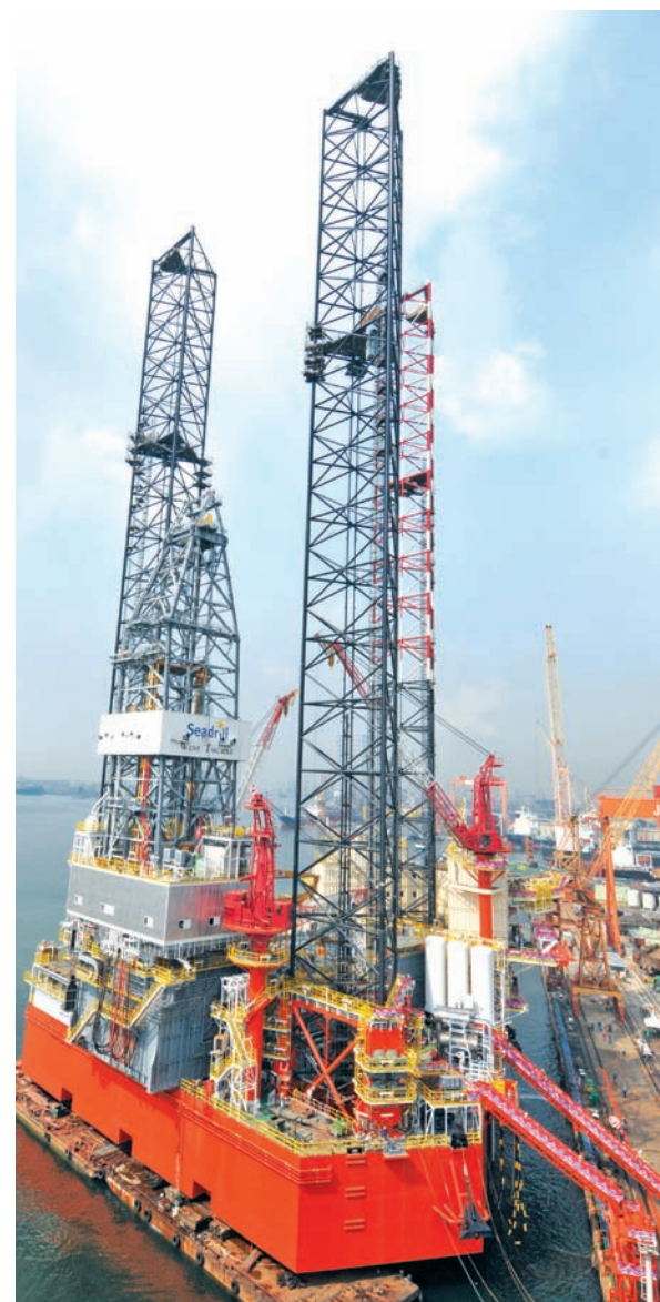
West Tucana, the first of two F&G JU2000E jack-up rigs for Seadrill, under construction at Jurong Shipyard.
