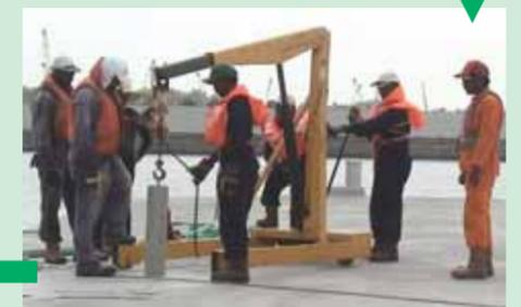
8. Installation of connector pins to join the pontoons.
